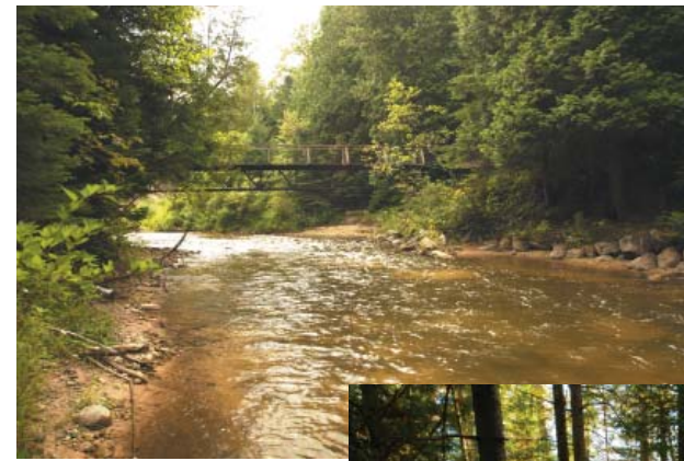
The bridge over the Pigeon River in front of the Andreae Preserve cabin.
